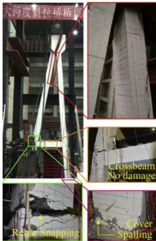
Fig.2 The deformation and local damage to the test model
