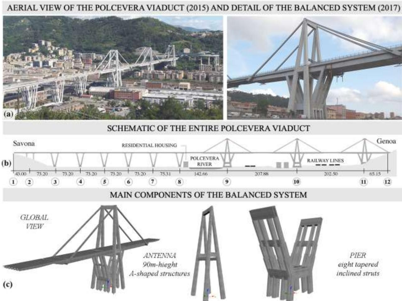
Fig. 2 – (a) Aerial photo of the bridge (left) and of a balanced system (right), (b) viaduct schematization and (c) main components of the balanced system, designed by Morandi [1]
