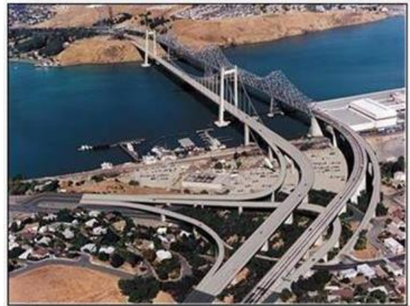
Figure 2. Aerial View looking towards Sacramento of the New Carquinez Bridge
