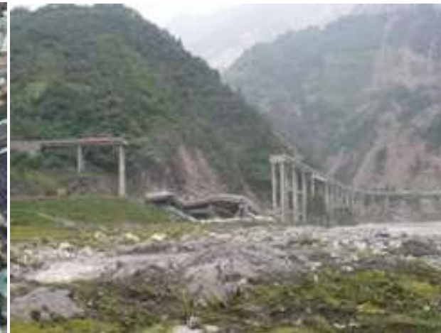
Baihua Bridge Wenchuan Earthquake 2008
