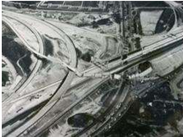
Separate bridge San Francisco earthquake 1971
