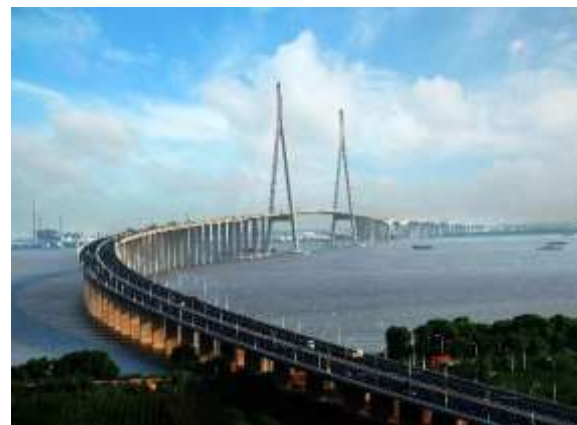
Su Tong Yangtze River Bridge 32.4 km, China, 2008
