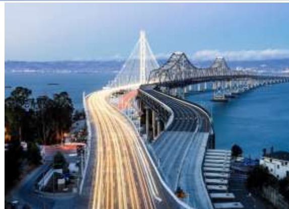
San Francisco-Oakland Bay Bridge USA, 2013
