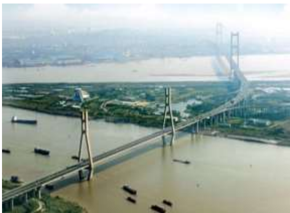
Runyang Bridge 35.66 km, China, 2004
