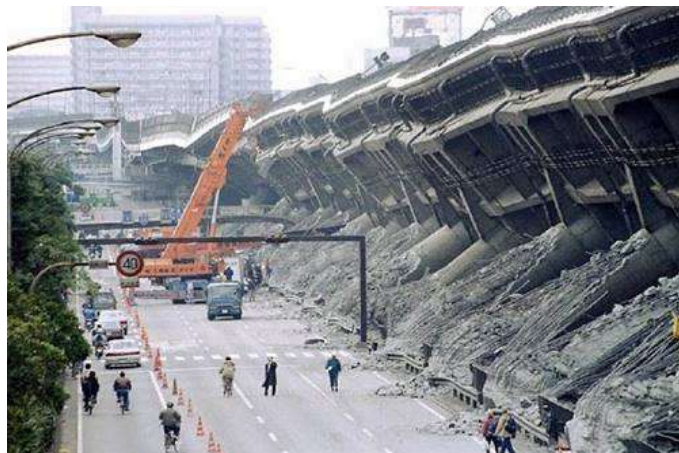
Kobe Earthquake, Japan, 1995
