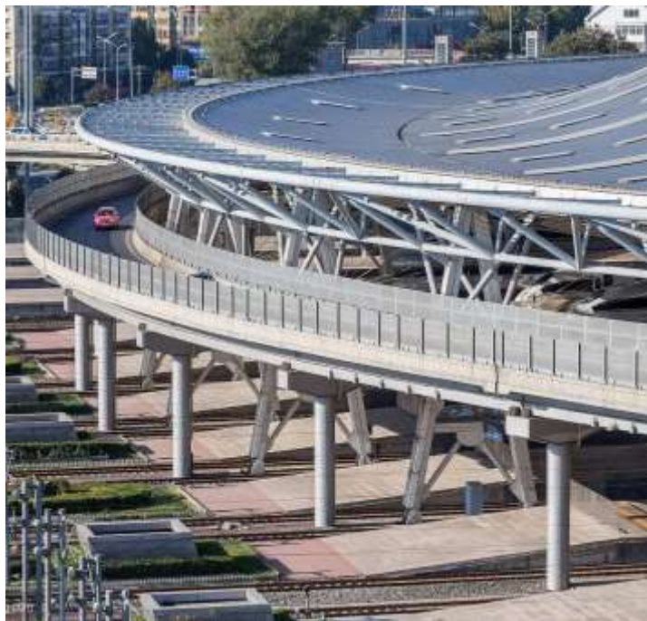
Beijing South Station Elevated Bridge
