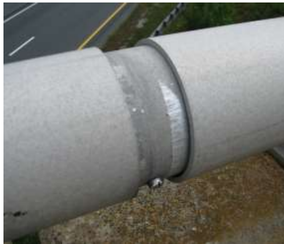
Figure 5. Displacement of Bridge Rail
