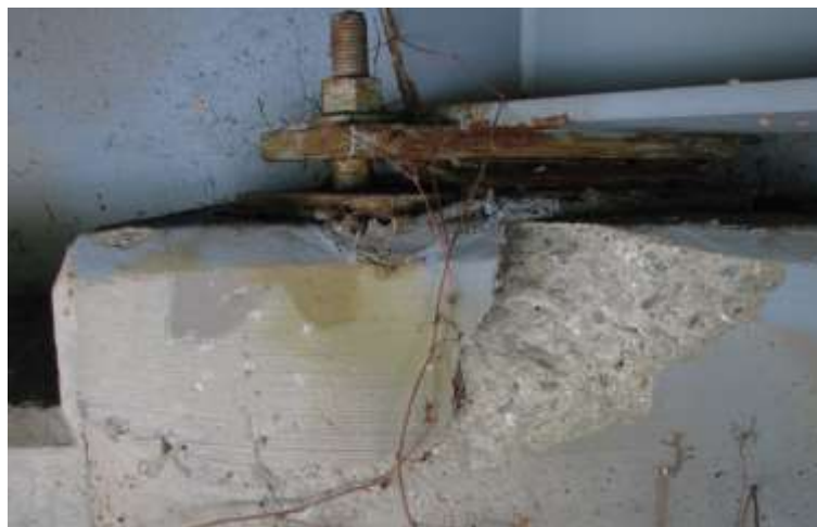
Figure 5. Displacement of Bridge Rail
