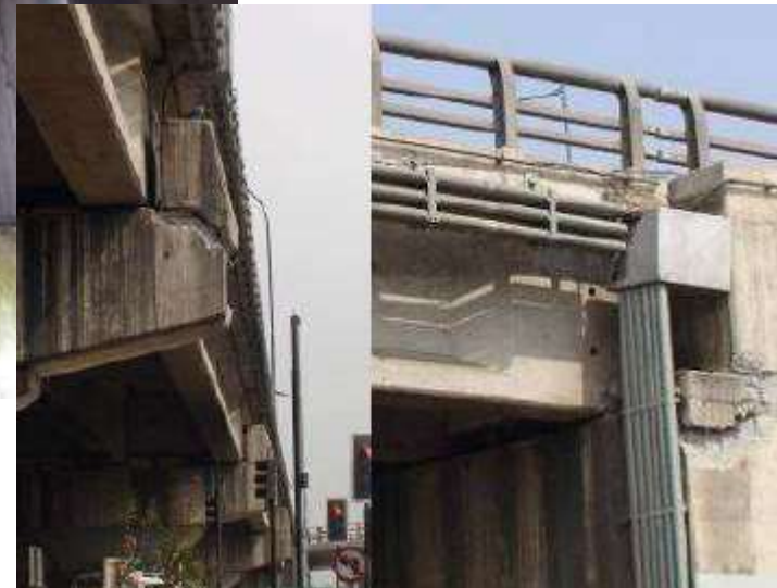
Llacolén bridge with internal concrete key (left)
