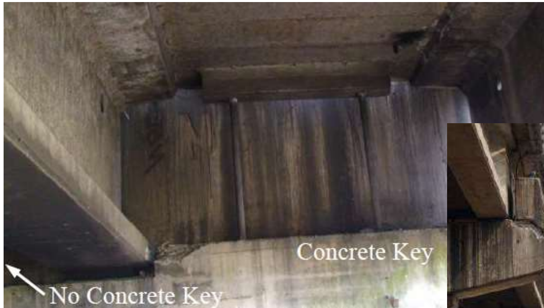
The Westbound Independencia bridge with external shear key (right)
